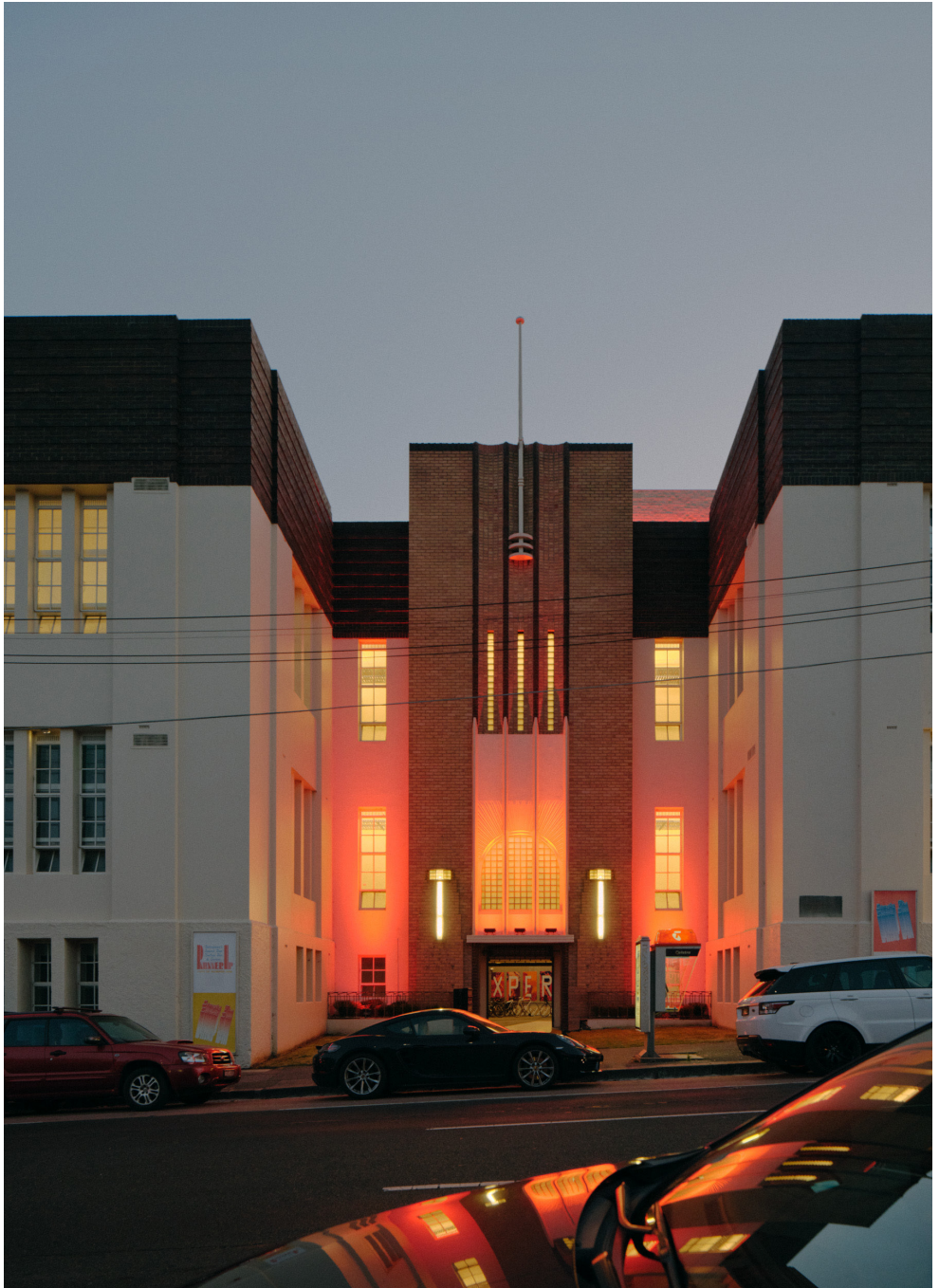
Johnst Street facade, by Tom Ross
